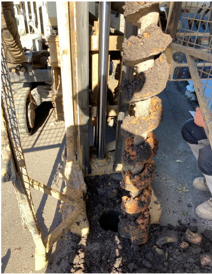
Residual soil encountered beneath fill in BH4a
