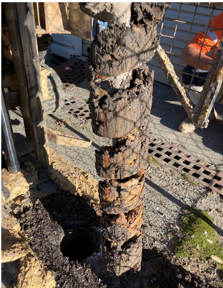
Residual soil encountered in BH6a
