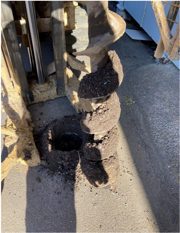
Fill material from BH4a was consistent with that observed in PSI borehole BH13
