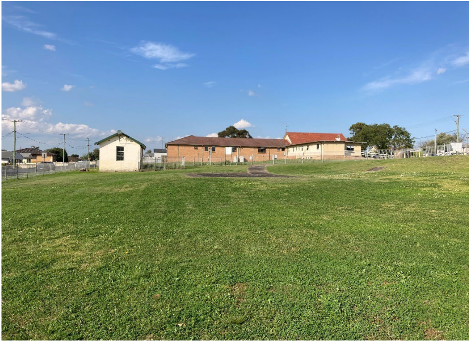
Looking Eastward from the northern grassed area. Areas of Fill are visible around and above Helicopter
