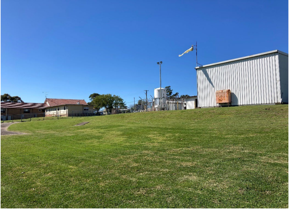
Liquid Oxygen Storage Tank and Yard Maintenance Shed at the top of a fill mound
