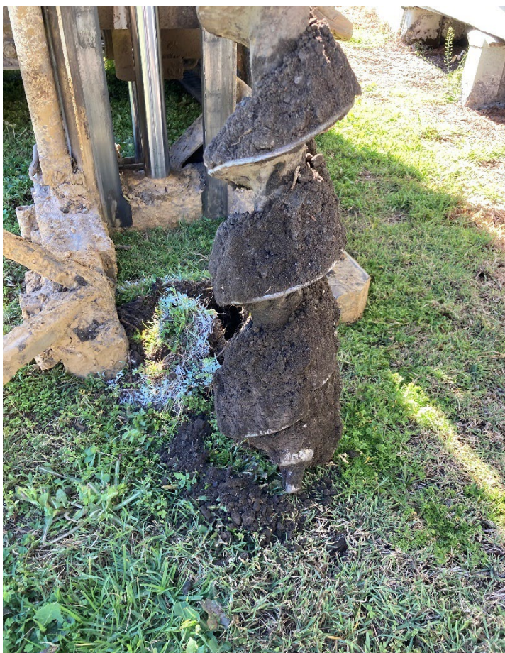
Fill material from BH5a at the rear of the former workshop buildings
