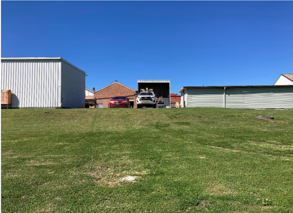
To the west of the Yard Maintenance Shed. The rear of the incinerator building is visible
